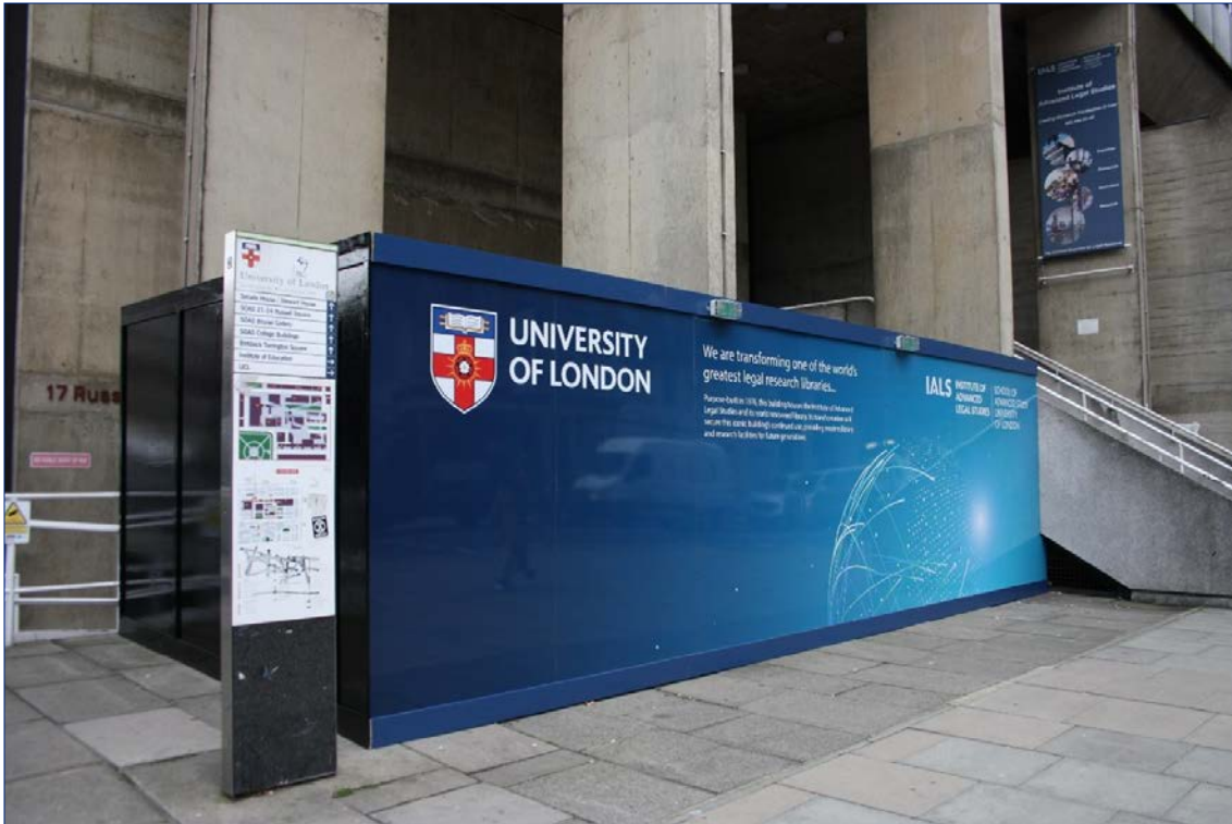
Mid-transformation: the current exterior of IALS
