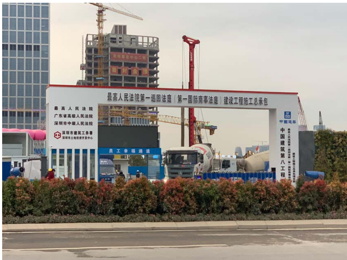
The CICC under construction
