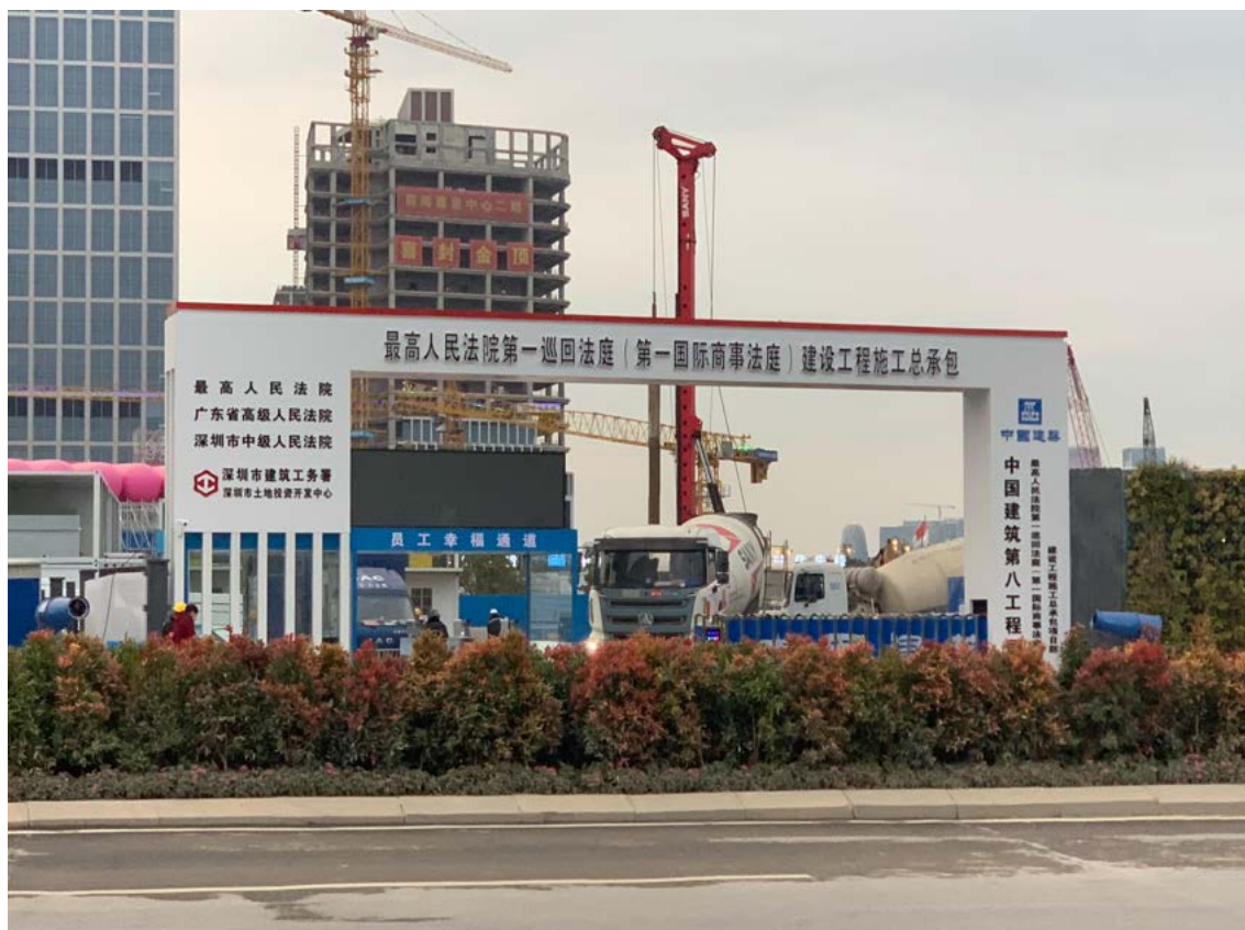
The CICC under construction
